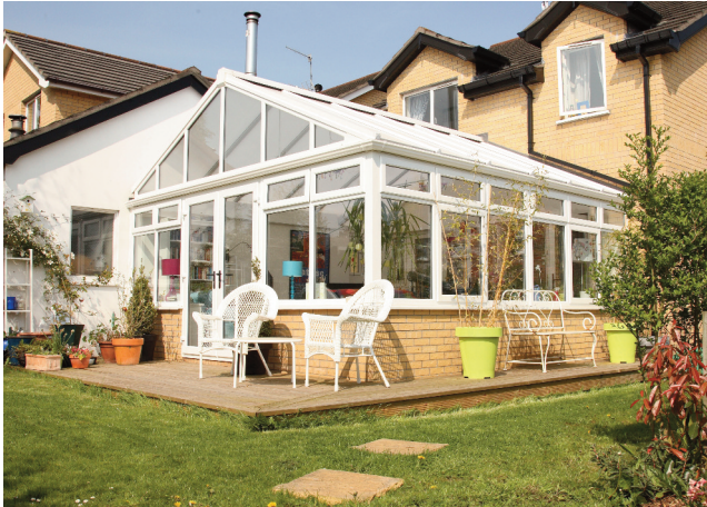
Gable fronted with finished brick. This conservatory connects the garage to the house.
