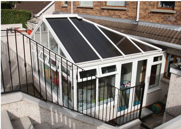
Approximately 120 tonnes of spoil removed to achieve this conservatory.
