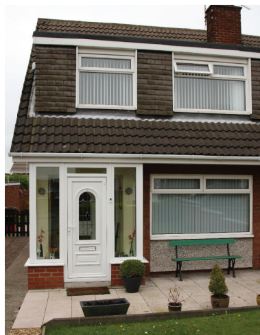
This porche uses the roof detail of the house, so it is cost effective.
