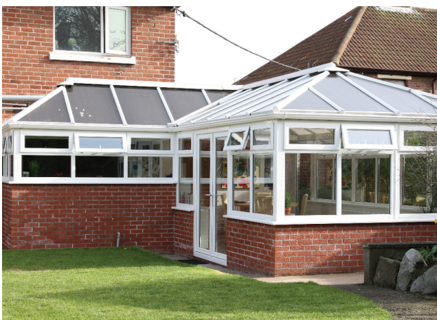
Two different wall heights in this one, the higher wall accommodates kitchen units.
