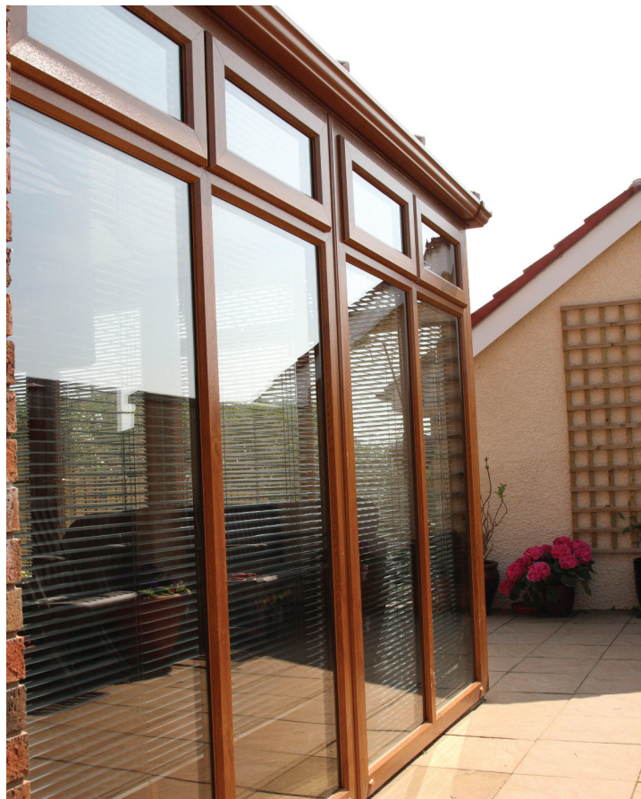
Although it doesn't look it there was approximately 10 tonnes of spoil removed on this particular conservatory for foundation and insulated sandwich type floor.
